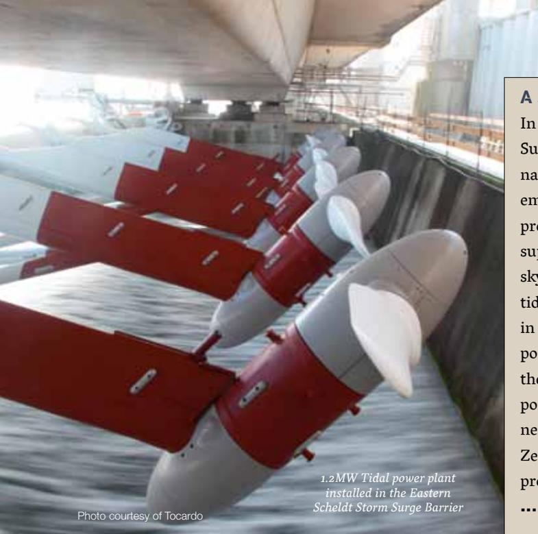
1.2MW Tidal power plant installed in the Eastern Scheldt Storm Surge Barrier
